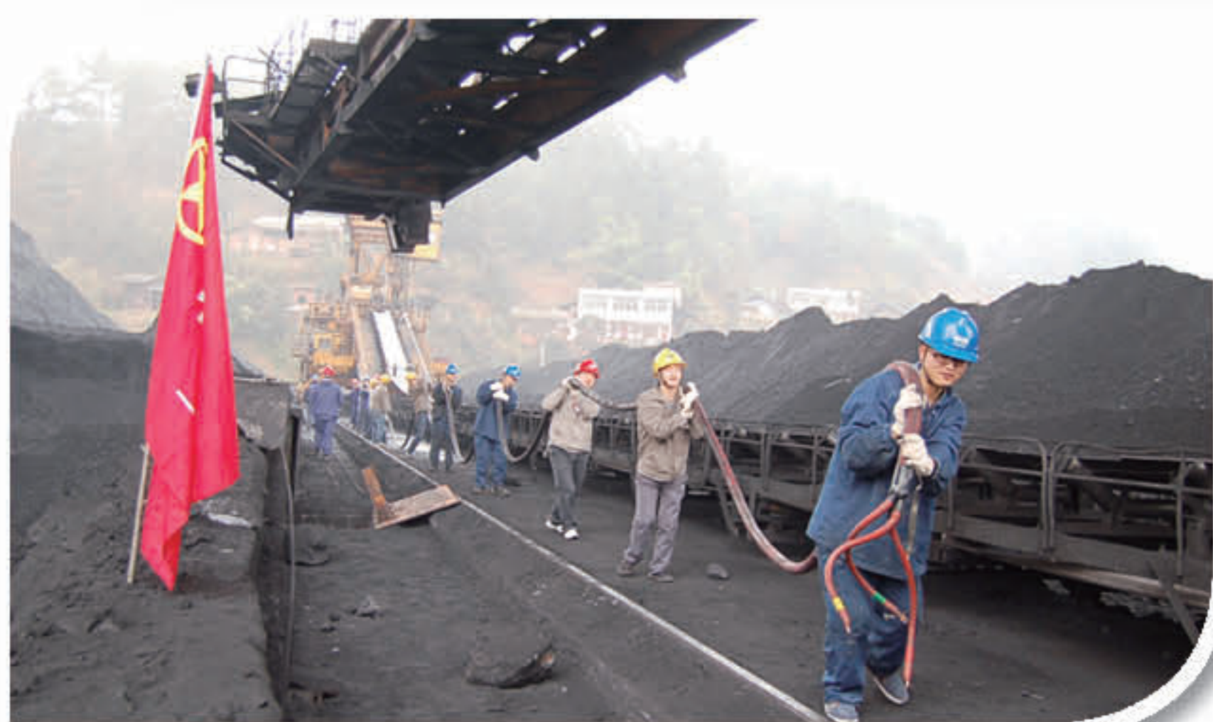
习水电厂青年突击队抢修斗轮机电缆
